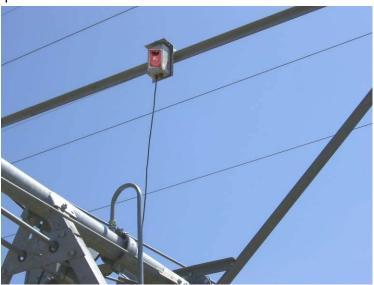
2. Mounted on the span pipe with the hose clamps (FC4893) supplied in the installation kit as shown in the pictures below.
